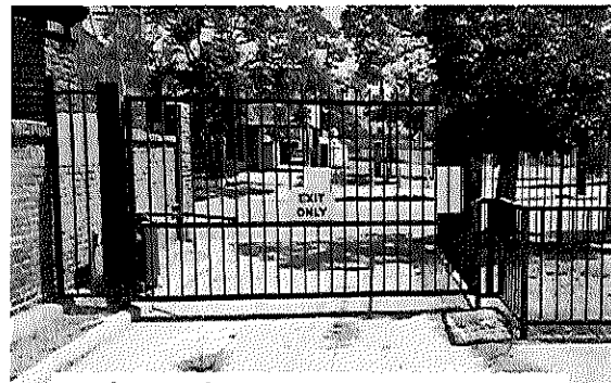
23rd St. Exit Gate
